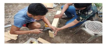
4. Assemble the parts of the frame using nail
